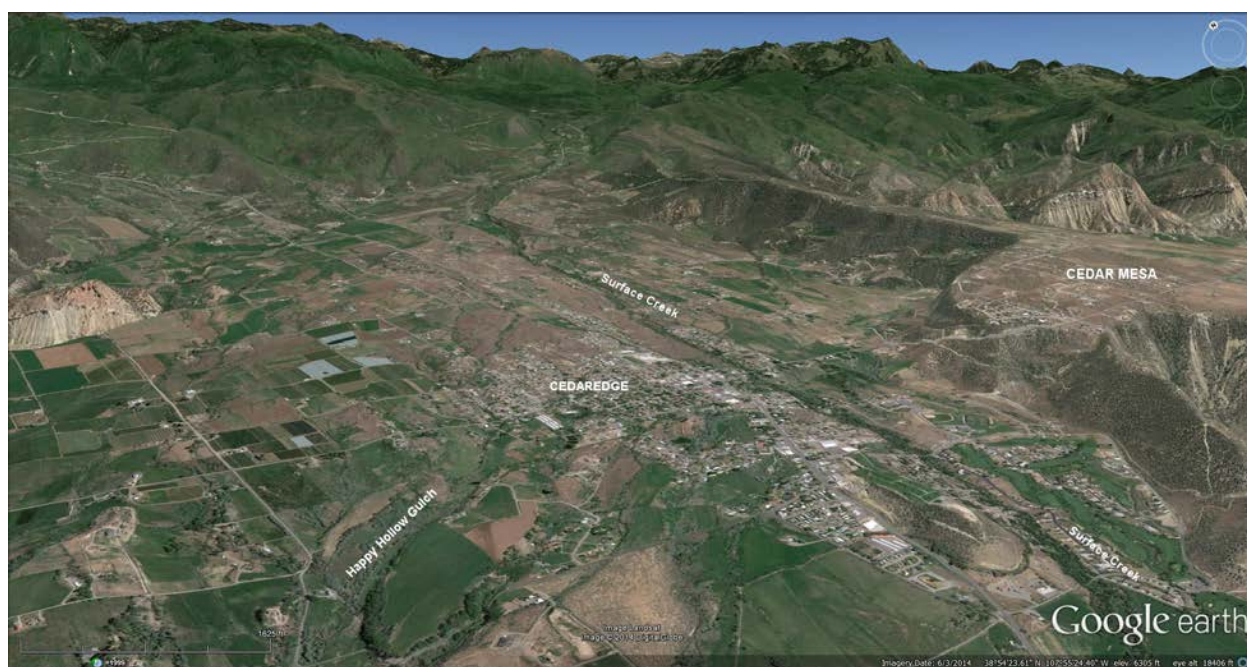
Figure 25b. Google Earth View of the Upper Section of the Valley Bottom Subsystem at Surface Creek, Looking Northeast. Note the Shale Outcroppings in the Lower Left and Right Indicative of Local Near-surface Bedrock.
